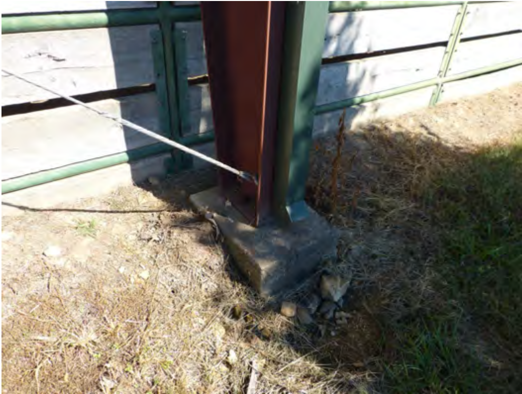
Figure 13 – Footing at girder G2R, Building C, South side.
