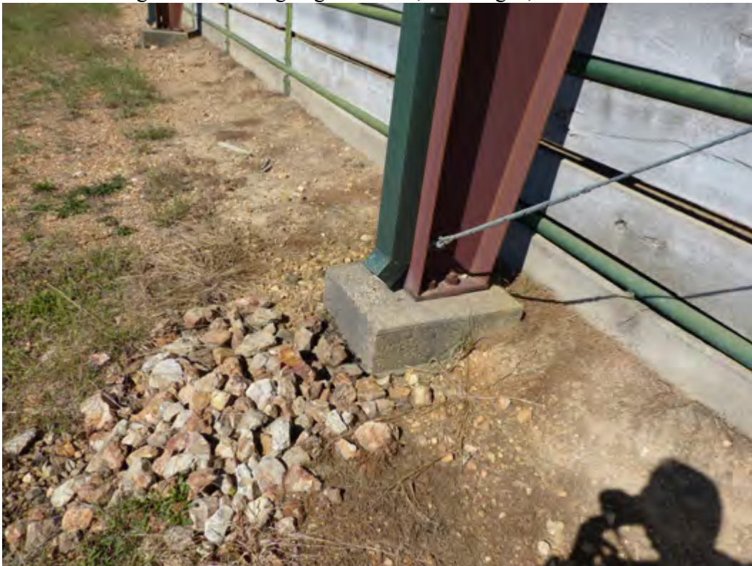
Figure 10 – Footing at girder G5R, Building C, South side.
