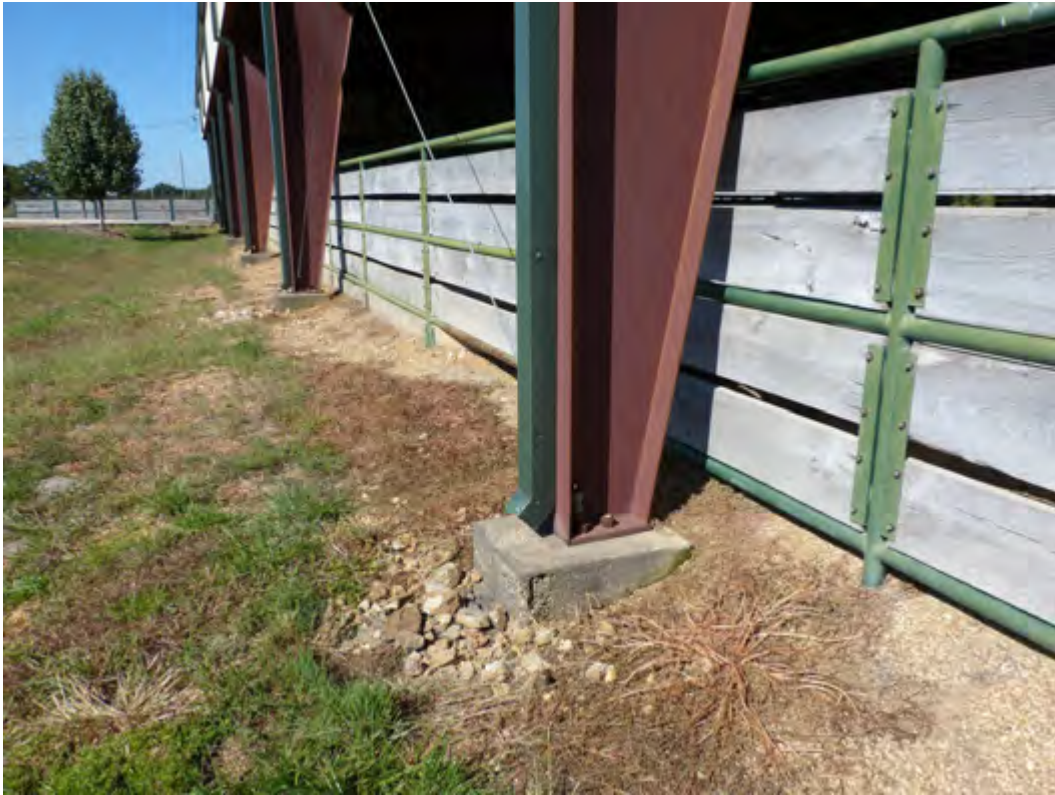
Figure 9 – Footing at girder G6R, Building C, South side.
