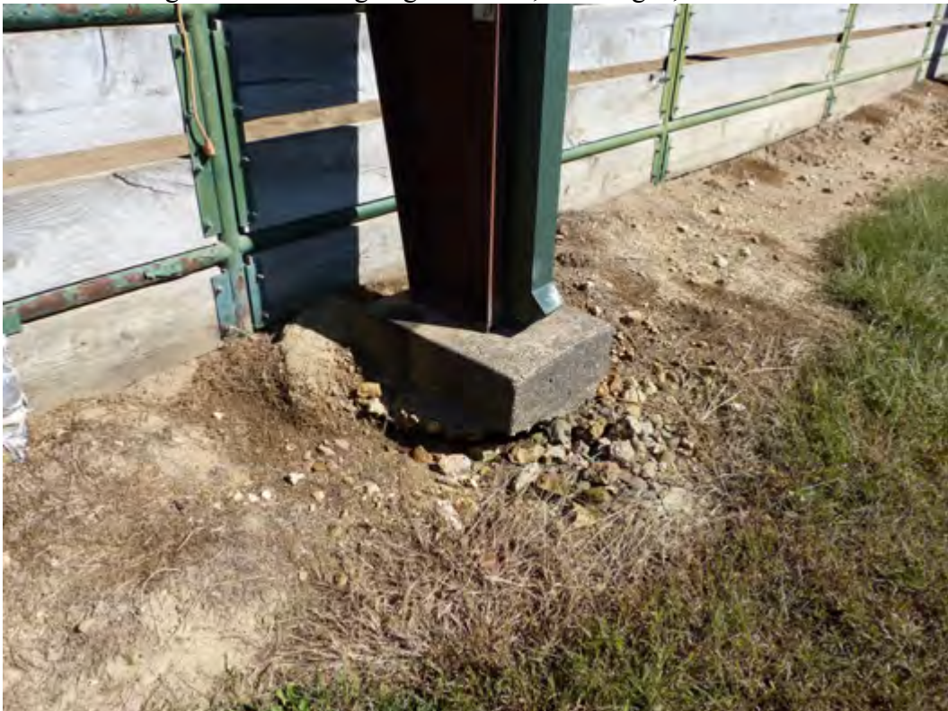
Figure 12 – Footing at girder G3R, Building C, South side.
