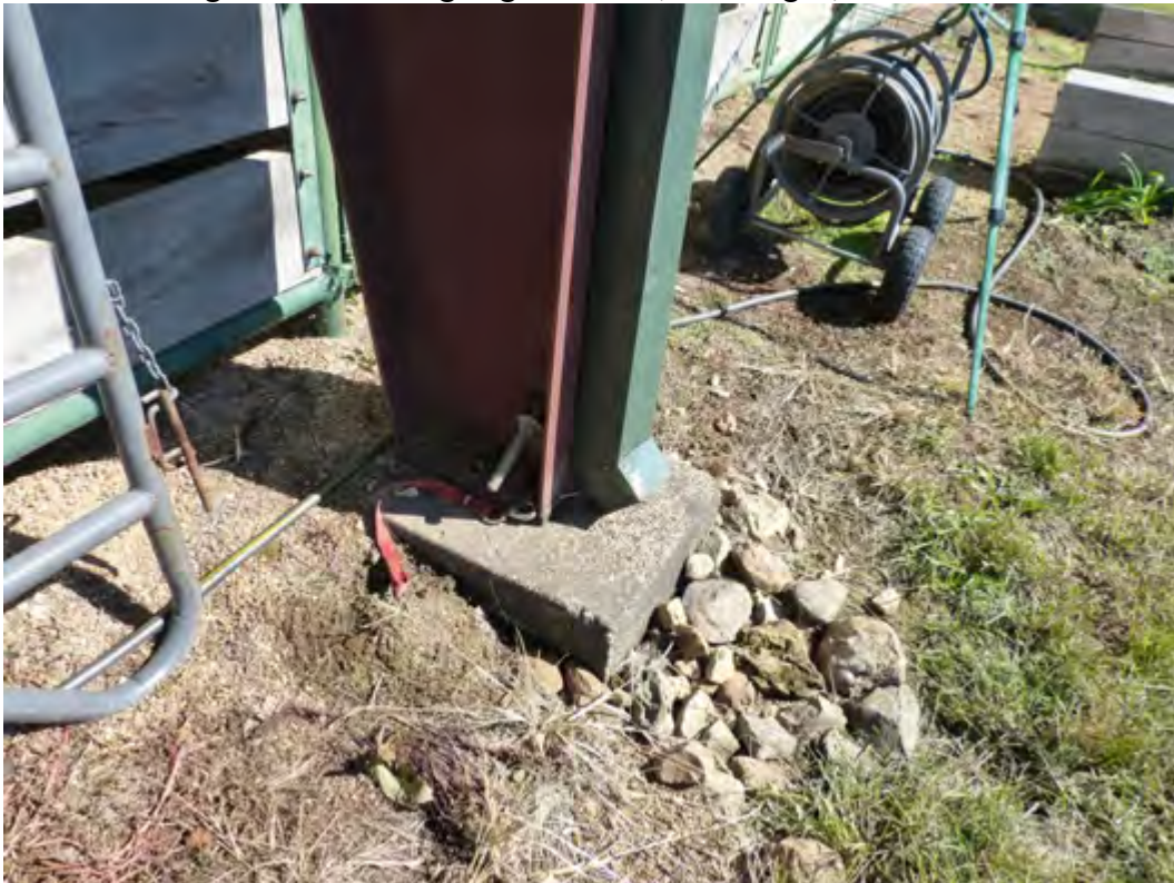
Figure 14 – Footing at girder G1R, Building C, South side.
