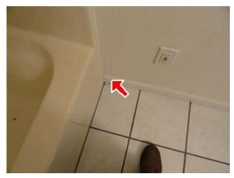
13.0 Picture 23 - Small tile crack
