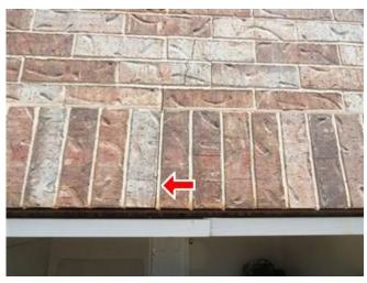
13.0 Picture 18 - Brick cracked over garage door
