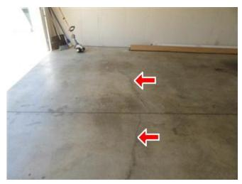
13.0 Picture 5 - Typical settlement/shrinkage cracks
