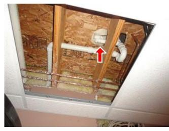
13.0 Picture 27 - Water stained tile from hydro tub drain leak (active)
