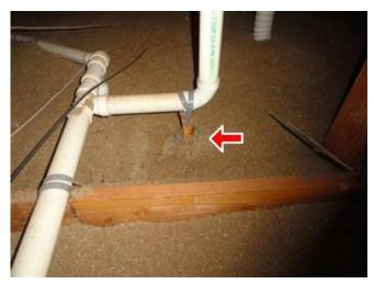
13.0 Picture 35 - Evidence of water leak at sewer vent pipe
