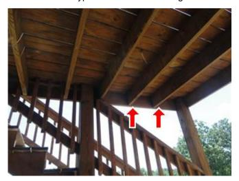
13.0 Picture 7 - Missing metal joist hangers
