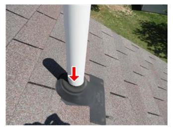
13.0 Picture 13 - Sewer vent boot needs replaced
