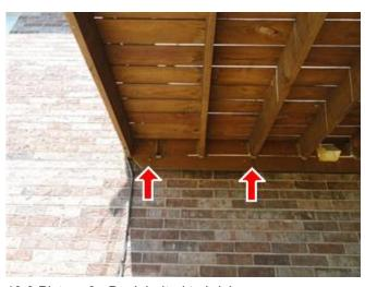
13.0 Picture 6 - Deck bolted to brick veneer
