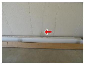
13.0 Picture 17 - Water stains from seepage at wall crack
