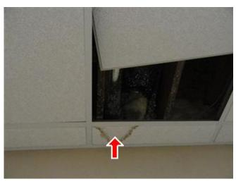
13.0 Picture 20 - Water stained tile from dryer vent condensation
