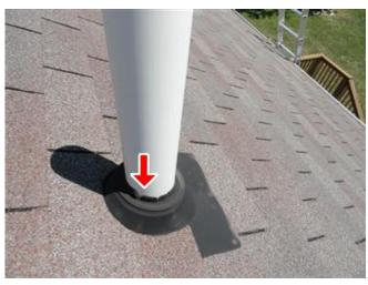
13.0 Picture 12 - Sewer vent boot needs replaced
