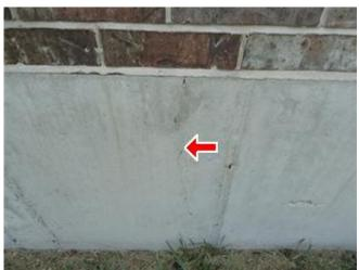
13.0 Picture 16 - Typical shrinkage crack
