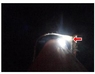
13.0 Picture 36 - Daylight showing at sewer vent boot
