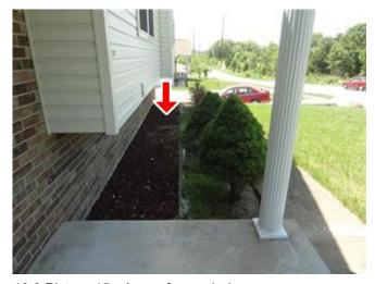
13.0 Picture 15 - Area of poor drainage
