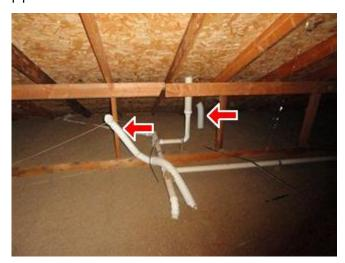
13.0 Picture 37 - Bathrooms vent into the attic
