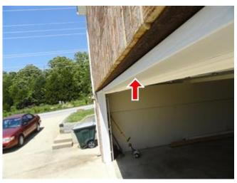
13.0 Picture 19 - Wall/beam over garage door has sagged 1/2 inch
