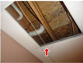
13.0 Picture 26 - Water stained tile from master bath toilet leak
